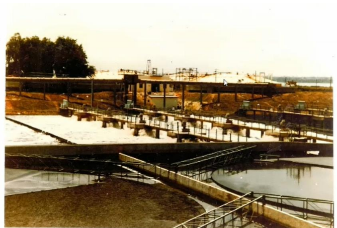
K & C VALLEY SEWAGE PLANT
